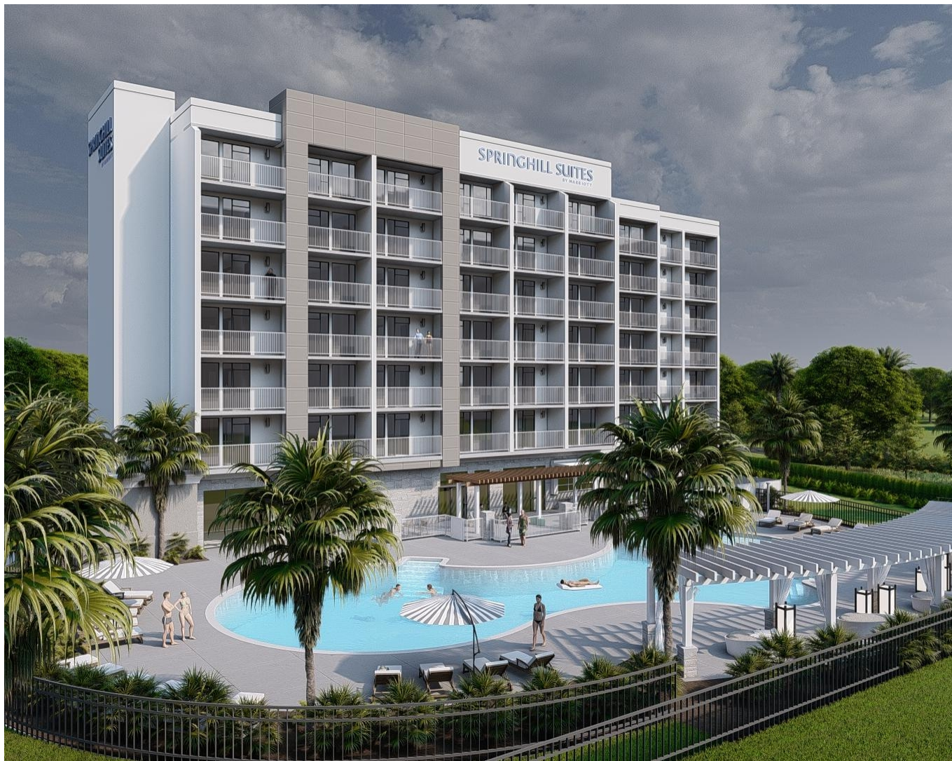
June 2023 South Elevation - AFTER
