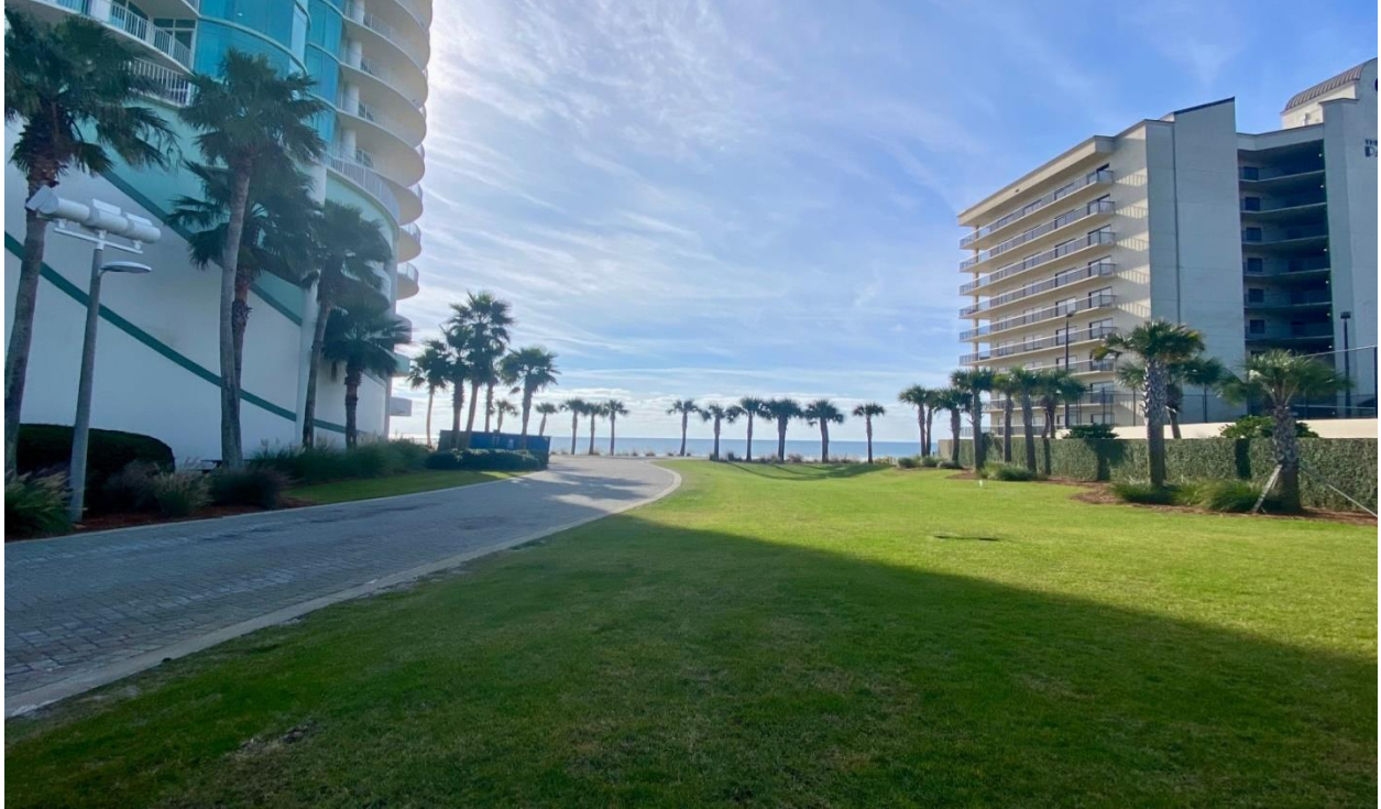
Site Visit, South Side (December 2023)
