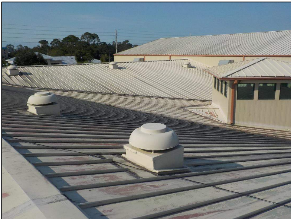
Overview photo of the North elevation roof
