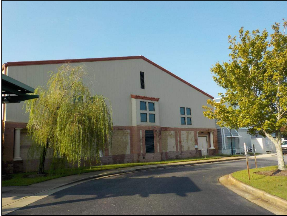
Overview photo of the Gym's North elevation
