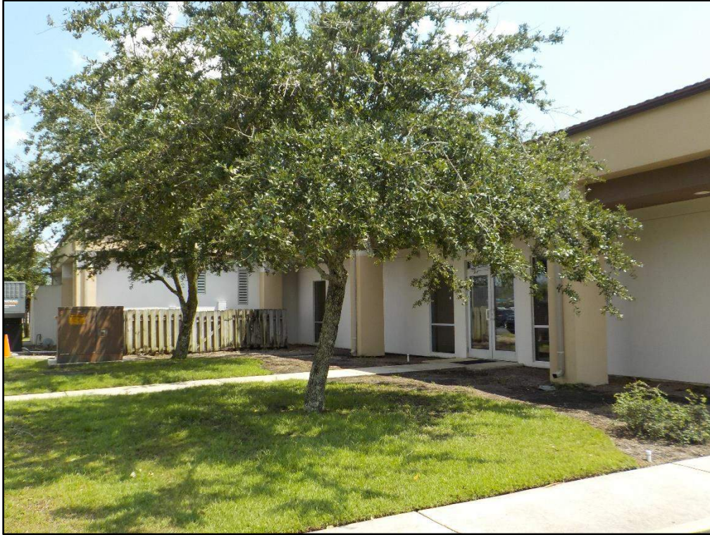
Overview of the North face West end of the building
