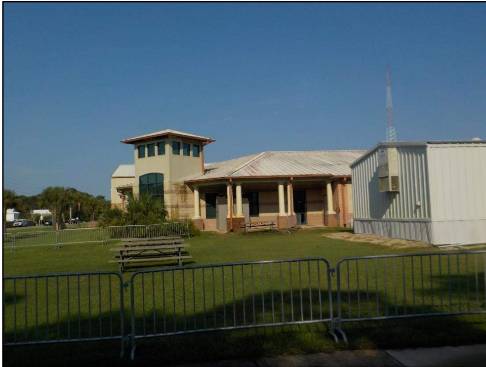
Overview photo of the Southeast elevation
