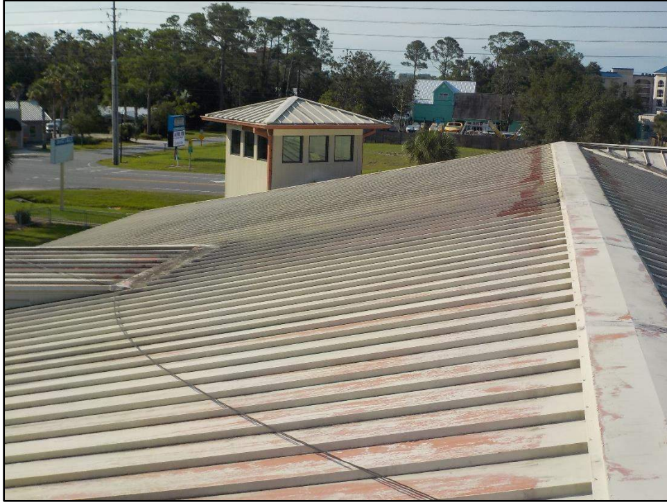
Overview photo of the East elevation roof
