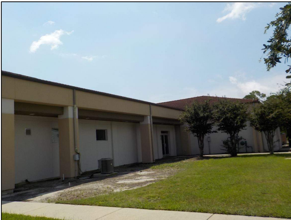
Overview of the North face East end of the building
