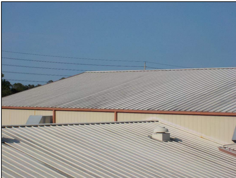
Overview photo of the Gym's East elevation roof
