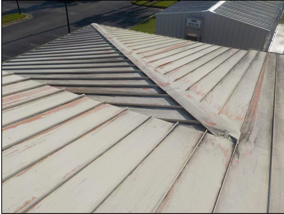
Overview photo of the North East Corner of the roof
