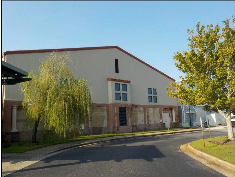
Overview photo of the Gym's North elevation
