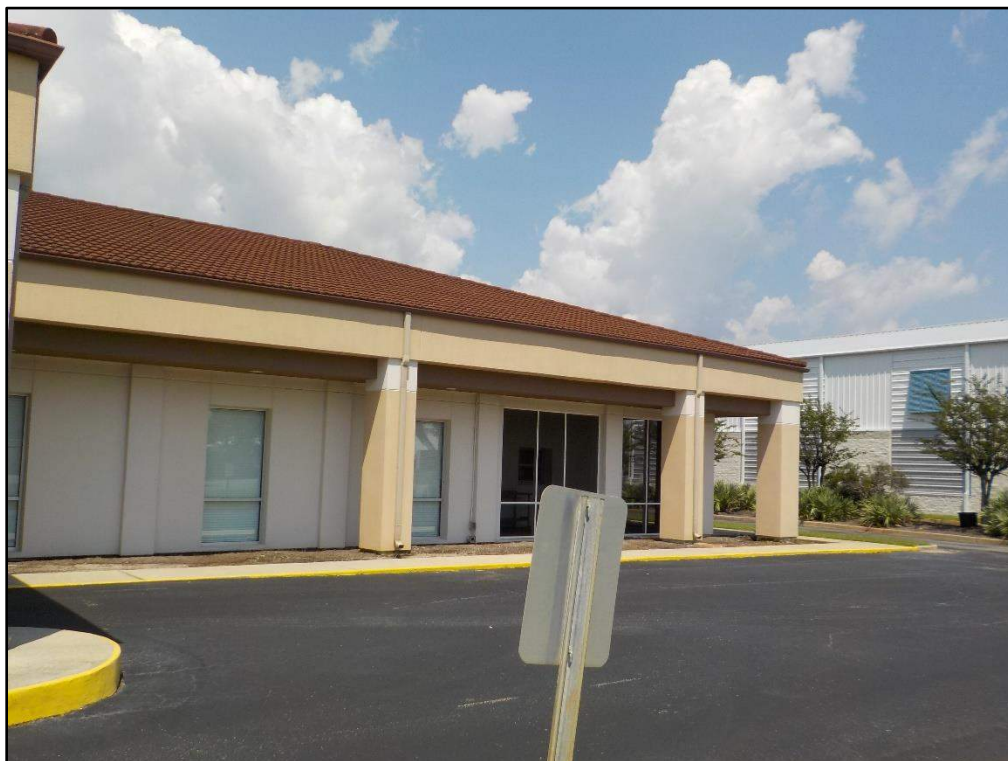
Overview of the South face East end of the building
