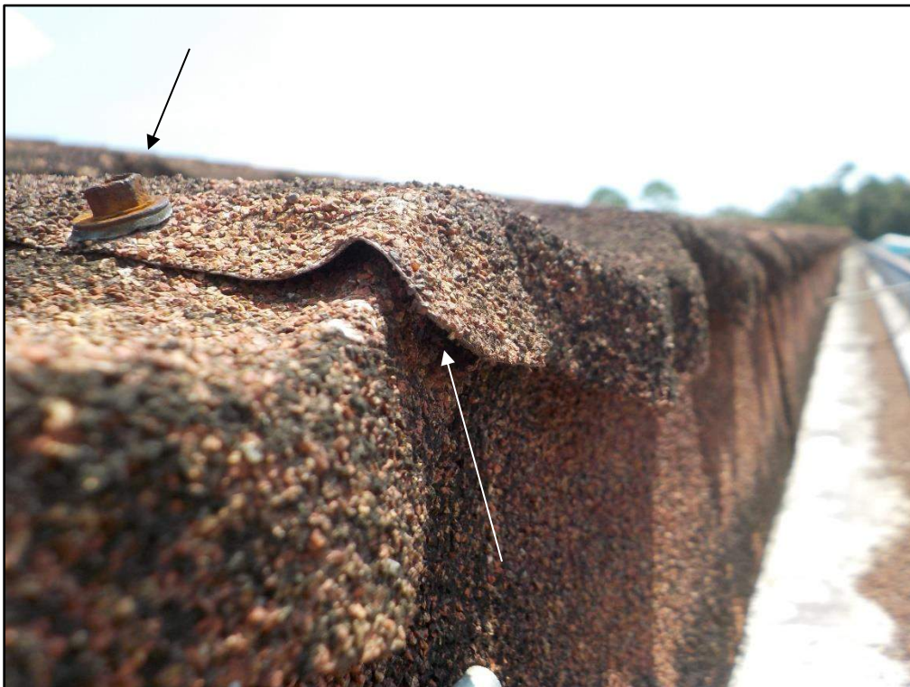
Fastener and thickness of material indicates metal r-panel
