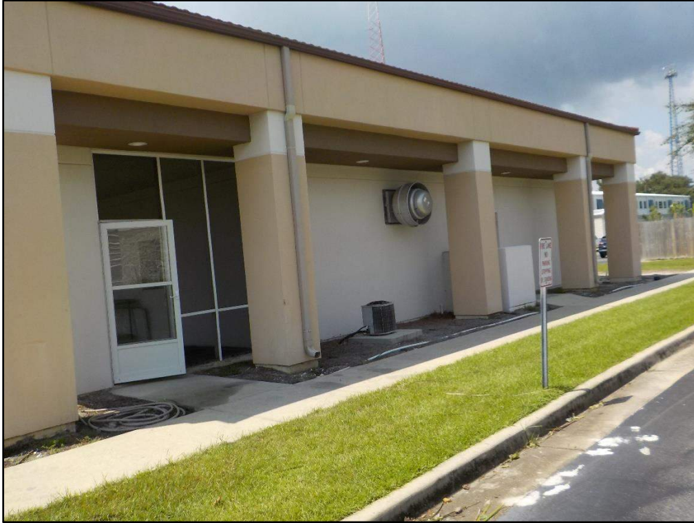
Overview of the East face wall of the building
