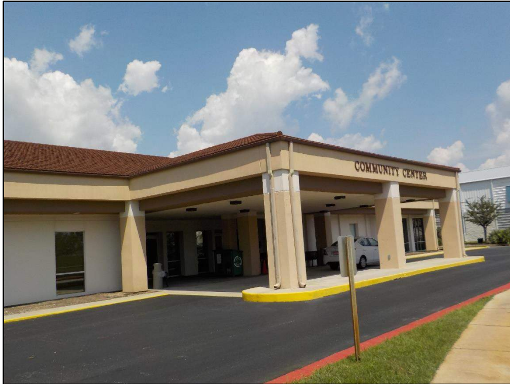
Overview of the South (front) Face of the building
