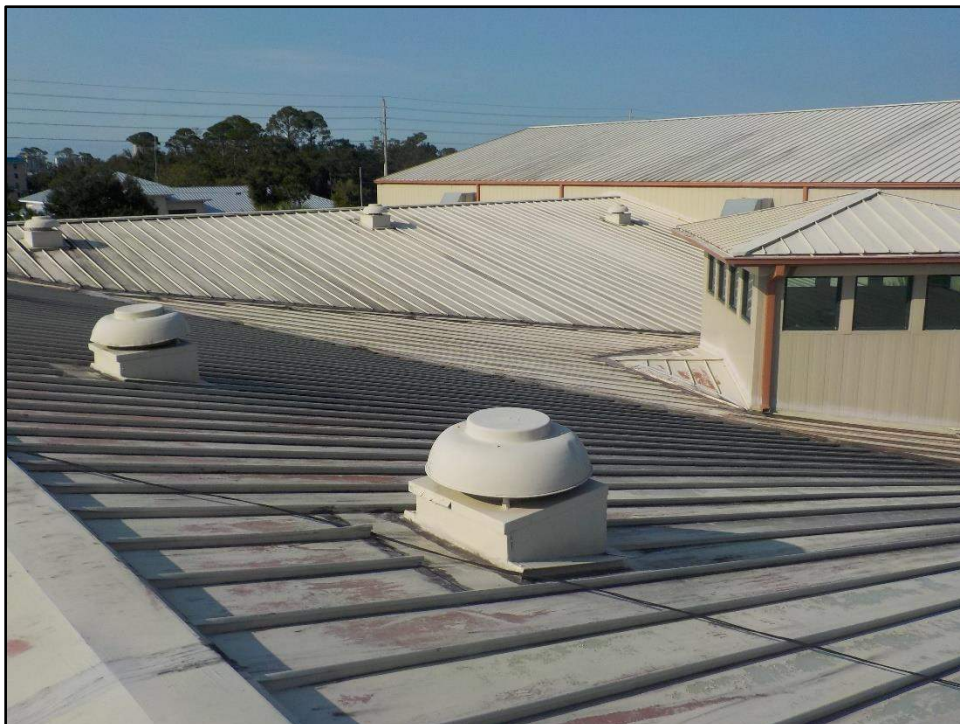
Overview photo of the North elevation roof
