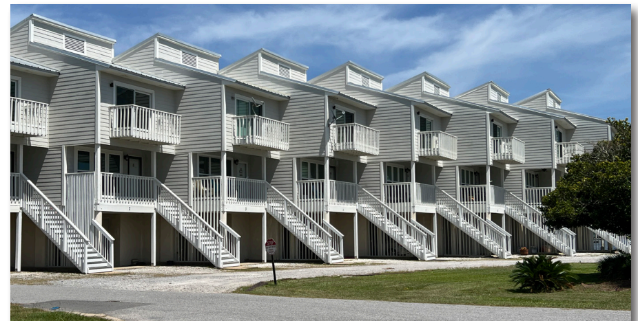
This housing development on Garrett Lane and fronting Cotton Bayou is significantly more dense than the adjacent single-family detached houses.
