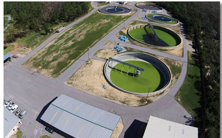
Operated by Orange Beach Utilities, this sewage treatment plant is located on the northeast corner of Powerline Road and Gulf Oak Ridge, just west of the Orange Beach Sportsplex. Source: City of Orange Beach
